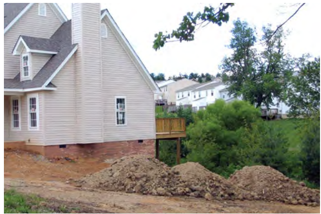
Figure 6.12. Stockpile topsoil prior to construction for later distribution before turf and landscape planting.
