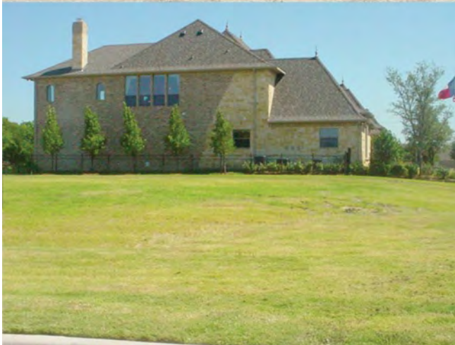
Figure 9.1. Ramifications of poor soil quality. Upper: Poor soil preparation. Lower: Poor turf establishment.
