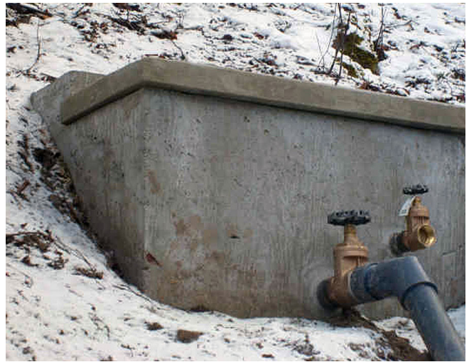
Figure 2. A properly sealed spring box will prevent surface water, insects and small animals from gaining access to the spring. Source: http://aquariuspump.com/springbox.aspx .
