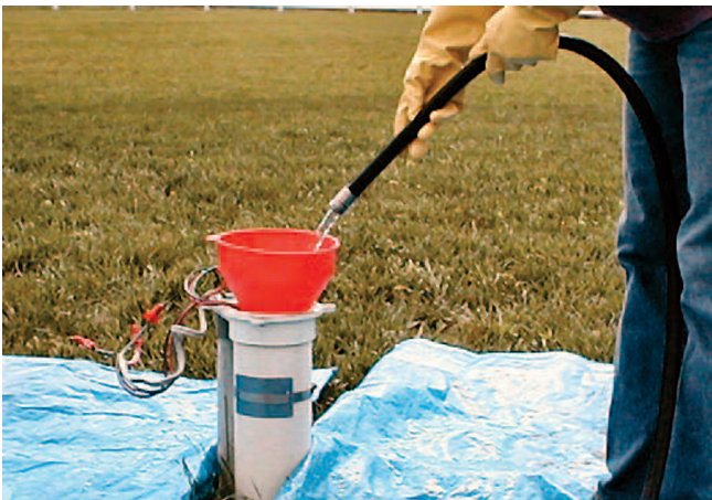
Figure 2. Circulate water in the well and wash down the inside of the casing. Source: Minnesota Department of Health. www.health.state.mn.us/divs/eh/wells/waterquality/disinfection.pdf .
