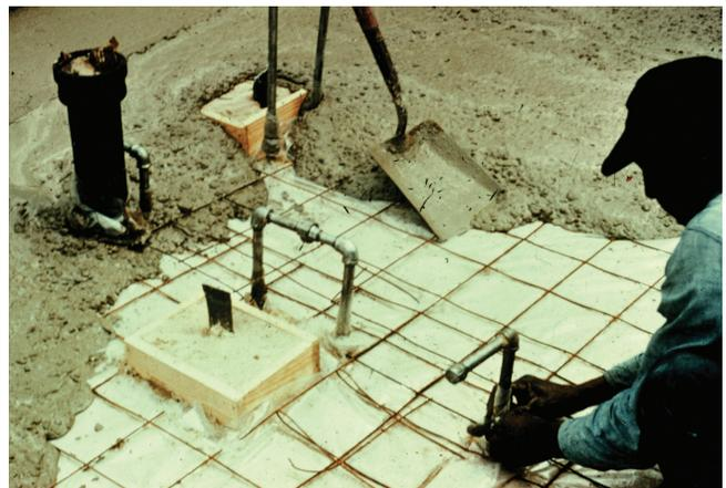
Form boards not removed after the slab is poured.
